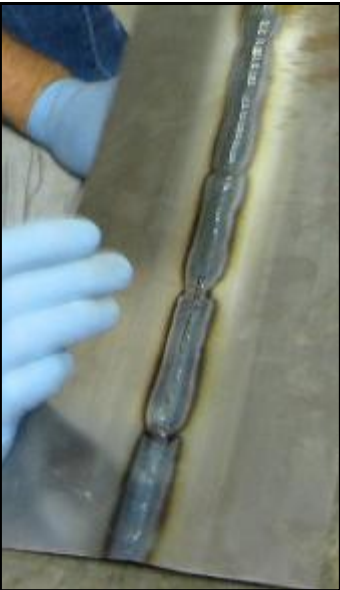
Below: TIG welds and far below: Removing the metal tape on the back-side of a TIG weld.
